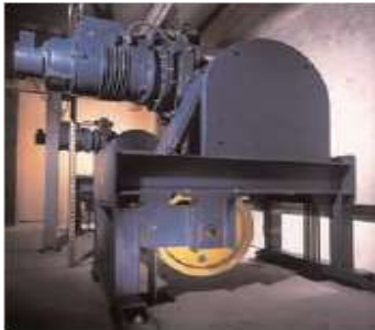
Gambar 2. Geared Elevator
