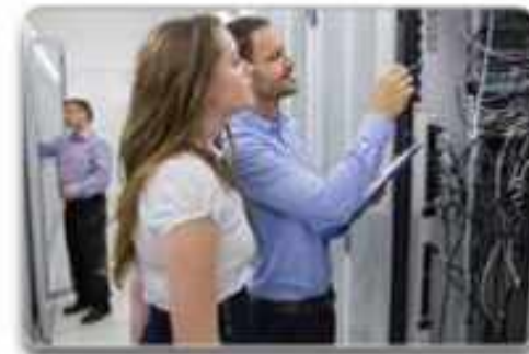
Installations must be inspected for damage.
